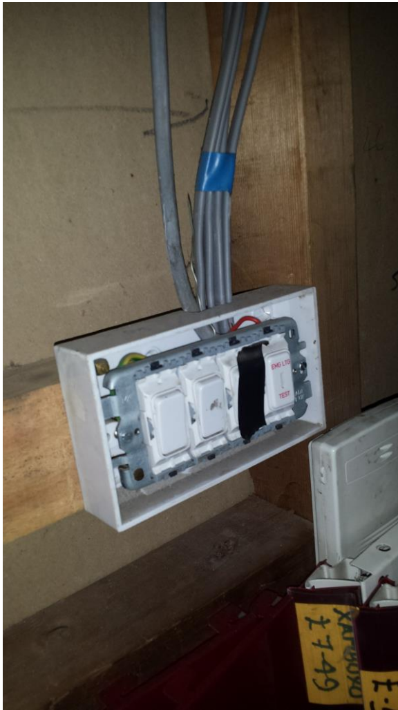
Picture on the left shows a bank of switches with the front casing removed. The picture on the right shows exposed live parts. A degree of protection should be provided so this contravenes Wiring Regulations 2008.
